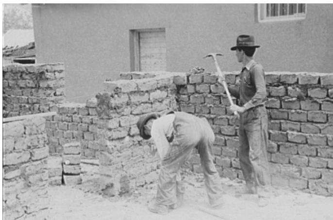
Constructing an adobe building, Penasco, New Mexico. Workers using an informal labor plan.
